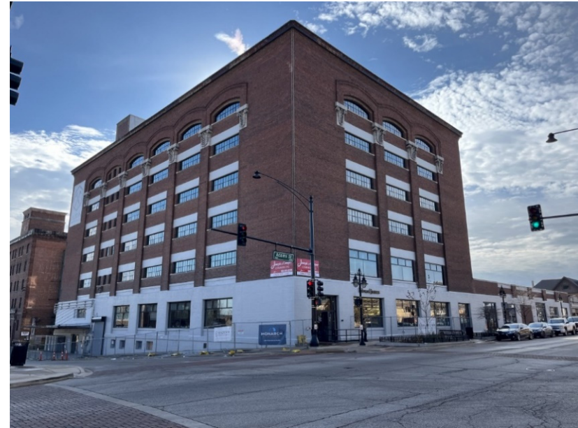
Adams and Oak (Under Construction)
