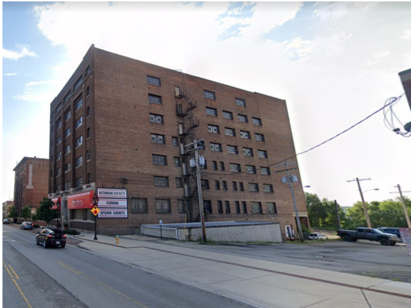
812 Lofts (Under Construction)
