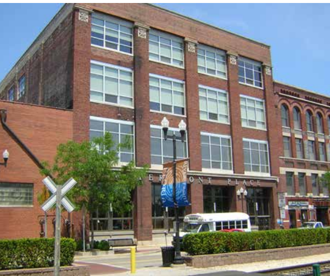
Lofts at Waterfront Place
