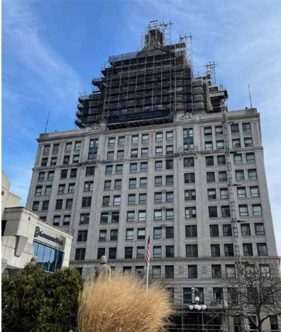
Peoria's second-tallest building is, for the moment, not quite as tall. Workers doing extensive repairs to the terra cotta façade of the building have removed many pieces, including elaborate panels at the very top of the tower. Many of them are spread out in a vacant office on the 10th floor of the 17-floor building.
